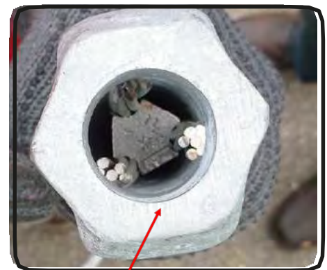
Correct Installation of Wedge
