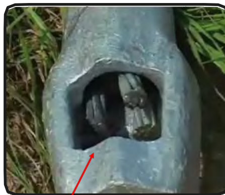
Correct Installation of Wedge
