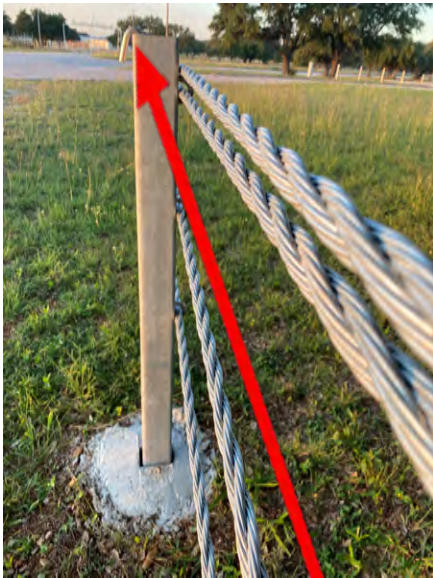
Installed Hairpin and Lockplate
