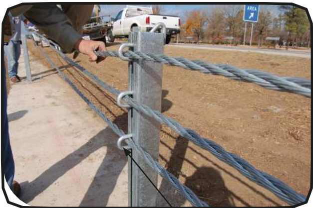
Installed Hairpin and Lockplate
